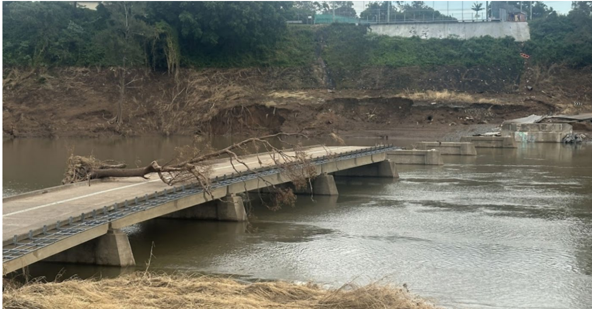
FIGURE 9 - THE BIGHT BRIDGE LINKING WINGHAM WITH TINONEE REMAINS OUT AND IS PLANNED FOR REPLACEMENT. NOTE THE SIGNIFICANT BANK EROSION ON THE FAR BANK
