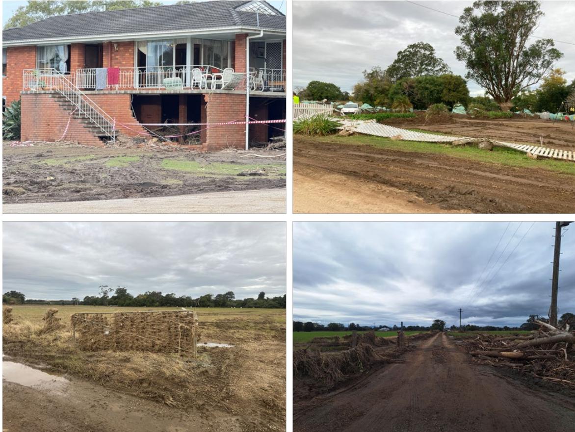
FIGURE 8 - GLENTHORNE ON THE OPPOSITE (SOUTHERN) BANK OF THE MANNING RIVER FROM THE TAREE CBD WHERE VAST AMOUNTS OF VEGETATION, MOTOR VEHICLES AND FARMING DEBRIS WERE DEPOSITED. (CLOCKWISE FROM TOP LEFT) (A) WALL COLLAPSED FROM THE FORCE OF WATER AND DEBRIS (NOTE LOGS DEPOSITED INSIDE GROUND FLOOR) (B) FENCE TORN DOWN, VEHICLES WASHED INTO PADDOCKS AND HUNDREDS OF ROUND HAY BALES STREWN ACROSS THE LANDSCAPE, (C & D) HUGE LOGS AND GRASS DEBRIS ALONG ROADWAY AND AMASSED IN FENCING AND GATES AS AN INDICATION OF WATER HEIGHT AND FORCE
