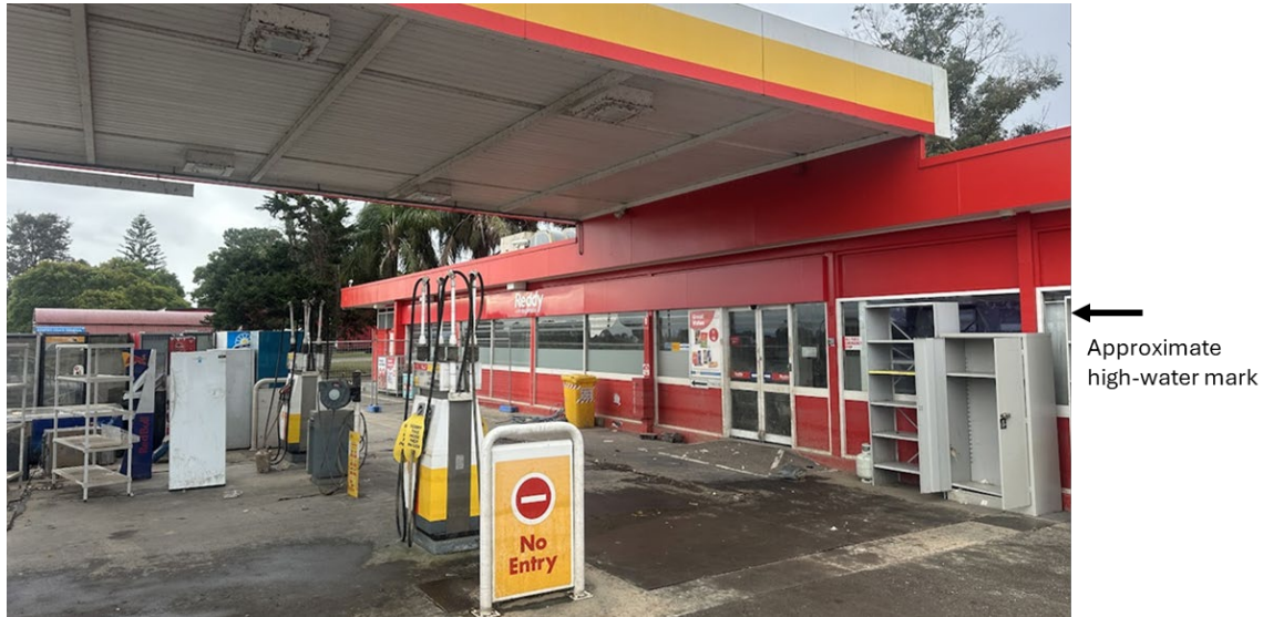
FIGURE 18 - A SERVICE STATION IN WEST KEMPSEY REMAINS CLOSED WITH THE REMNANTS OF FUEL BOWSERS, FRIDGES AND FREEZERS DESTROYED IN THE FLOOD BEHIND TAPE. FLOOD LEVEL AT THIS LOCATION WAS > 2 METRES
