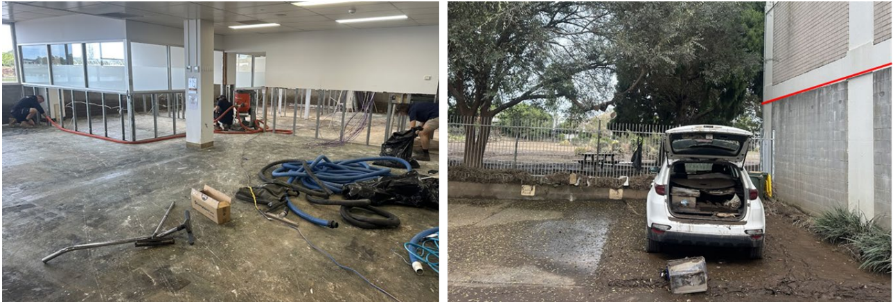
FIGURE 7 - FROM L- R: (A) CLEAN-UP CREWS CONTINUE STRIP OUT OF THE ENTIRE FIRST FLOOR OF THE EDUCATION CAMPUS. (B) VEHICLE ABANDONED IN THE QUICKLY RISING FLOOD WATER WHICH REACHED APPROXIMATELY 3 METRES IN THESE LOCATIONS (RED LINE) IN THE CAR PARK OF THE CAMPUS ADJACENT TO THE MANNING RIVER (LEFT) AND CBD (RIGHT)
