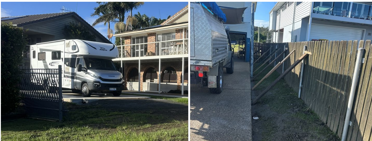
FIGURE 13 - EXPERIENCE WITH FLOODING IN 2021, THESE RESIDENTS ON SETTLEMENT POINT DRIVE IN PORT MACQUARIE HAVE INCREASED THEIR OWN PERSONAL RESILIENCE BY MAKING PREPARATIONS TO PROTECT PERSONAL PROPERTY. (IMAGE ON LEFT) - SHOWS A NEWLY CONSTRUCTED ELEVATED CONCRETE SLAB AND NEW MOTORHOME WHICH AVOIDED INUNDATION ON THIS OCCASION. (IMAGE ON RIGHT)-AFTER LOSING FENCES IN 2021, THIS RESIDENT HAS REINFORCED FENCES WITH TEMPORARY TIMBER BRACING AND GALVANISED STEEL POLES WITH CONCRETE FOOTINGS (IMAGE TAKEN FACING AWAY FROM RIVER)
