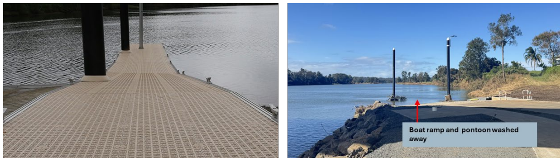
FIGURE 15 - FROM L-R, (L) THE BOAT RAMP AND PONTOON IN SITU AT THE ROCKS FERRY RESERVE PRIOR TO THE 2025 FLOOD (R) THE PONTOON AND RAMP WASHED AWAY
