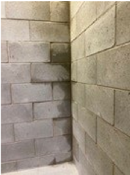
Figure 7: Water ingress through masonry walls
