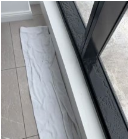
Figure 8: Wind driven rainwater ingress through window systems
