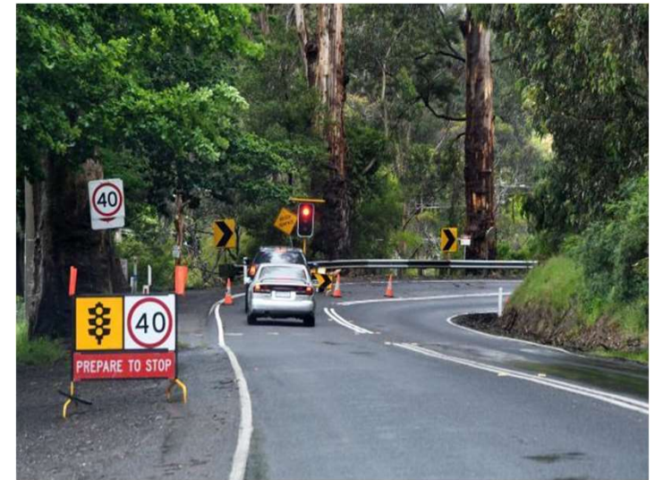
Temporary one lane operation following the landslip. Image credit: Stewart Chambers, Upper Yarra Mail
